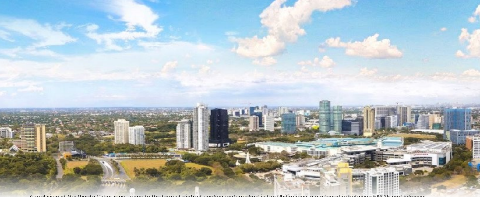
Aerial view of Northgate Cyberzone, home to the largest district cooling system plant in the Philippines, a partnership between ENGIE and Filinvest.
